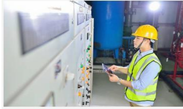
Figure-3.43: Preventive Maintenance Practice Courtesy: Image from freepik.com
