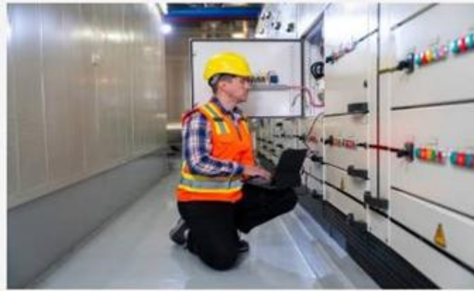
Figure-3.44: Corrective Maintenance Practice
