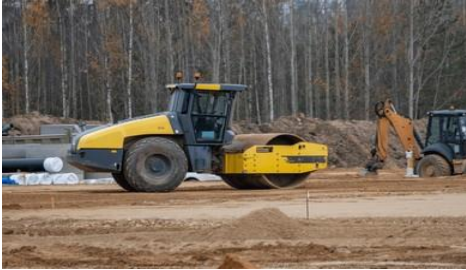
Figure 4.3 रोलिंगद्वारे मातीचे कॉम्पॅक्शन (Compaction of Soil by rolling)
