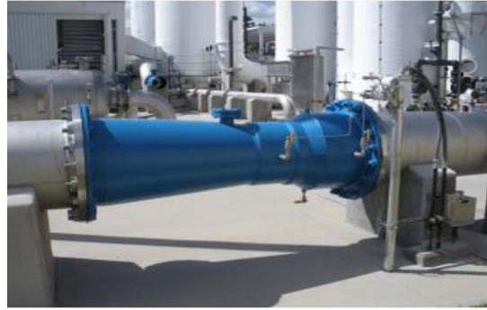
Fig 3.1 Venturimeter (www.indiamart.com)
